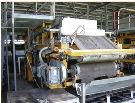
Figure 2. Current Belt Filter, producing 70 tonnes per day of 15% cake.
